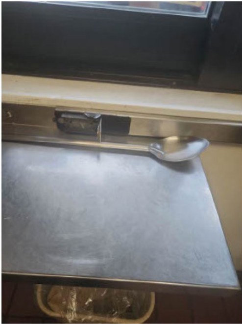
Spoon wedged under broken lock in drive-thru window
